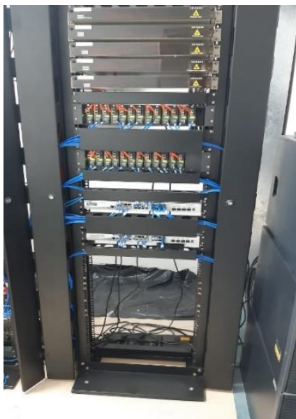
Figura 12 - Rack 1- Switch Core
